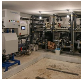
Space, lighting and clear equipment plumbing layout increase comfort, ease of service, while reducing maintenance errors and increasing energy and ergonomic efficiency.
